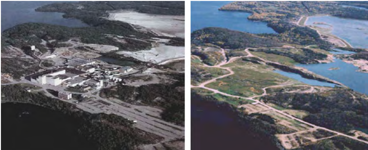
Plate 17: Aerial views of the Denison Mine before and after reclamation (from Canadian Nuclear Safety Council).
